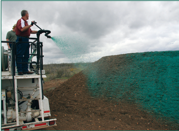
Figure 5. Hydroseeding.
